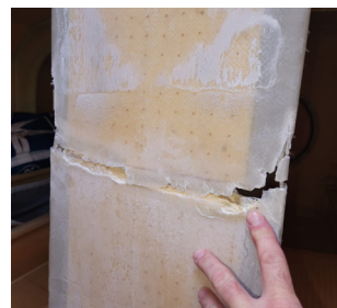
The damaged frame.
